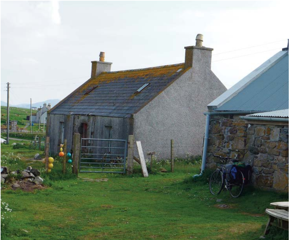
The old Croft House adjacent to the hostel is ready for restoration. Photograph by Peter Clarke.
